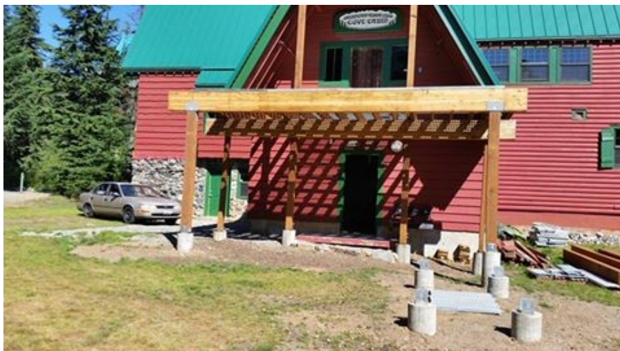
WAC Cabin 's new deck is taking shape
